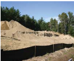
Proper Use of Silt Fence
