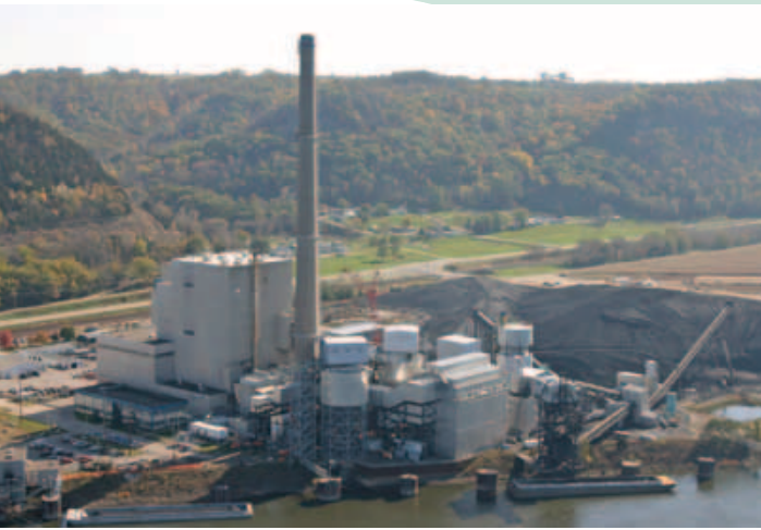
New emission control equipment, including the “baghouse” and scrubber system, can be seen in the foreground of Genoa Station #3.
